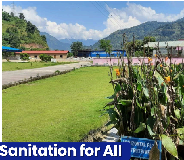
The before (L, October 2020) and after (R) picture of Fecal Sludge Treatment Plant (FSTP) in Waling Municipality, Nepal. JSR 2023 notes the growing need for well designed septic tanks and FSTPs. Both Photos: CWISAN/MuNASS
